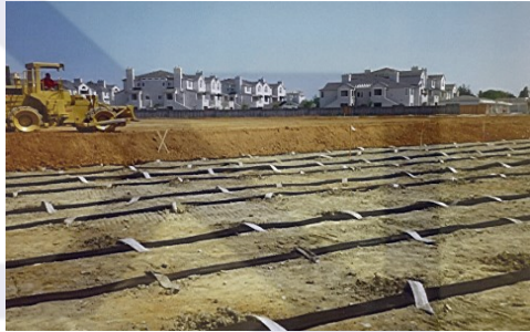
Lateral Strip Drains
